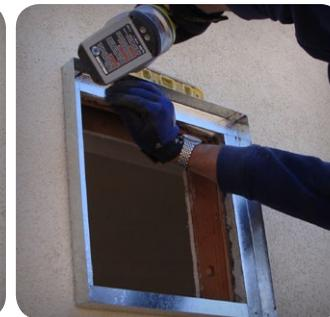
9. Place fan into the cut out area. Fasten the fan in each 4 corners to the vertical wood studs (see **Figure 2.3E**).
