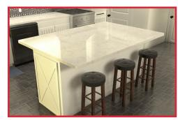
**6.** Check once again that the counter top is level. Once level, caulk around the brackets with clear silicone to hold your counter top securely.
