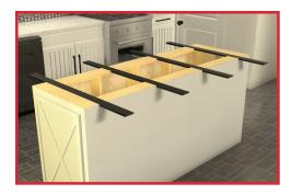
**2.** Rout or chisel a 2.5" wide by 0.5" deep pocket at each mark on both sides of the cabinet. This "pocket" will allow the bracket to sit flush with the top of the cabinet. (Make sure it is flush)
