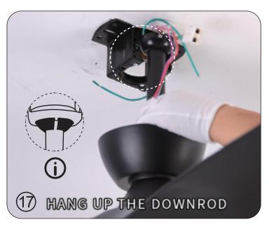
WARNING: Turn off the electric power during installation and making wire connection.
