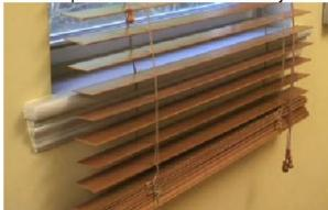
Step 2: Select the slat that is even with the window sill or slightly below it
