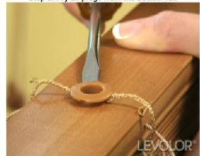
Step 6: Remove the bottom rail from the excess slats
