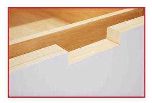
1. Mark 2"-4" from the outer edge of your cabinet for your first notch to be cut. Then set marks for the remaining brackets every 16"-20" apart. Rout or chisel out a 0.5" deep by 2.5" wide notch from the cabinet. Top of bracket should be flush with top of the cabinet.
