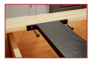
3. Once your brackets are in place and level, using the holes on the bracket as a guide, drill pilot holes into the top stretcher. Once pilot holes are made, drill the screws through the pilot holes, fastening the bracket to the stretcher.
