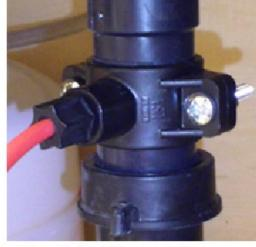
Fig. 5 Drain saddle
