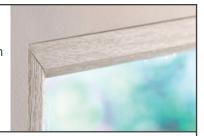
Measure the **inside** width & height of the door glass opening as shown below.
