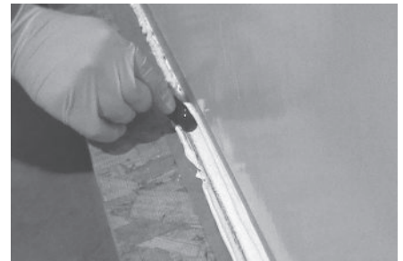
FIGURE 23: HORIZONTAL FINISH WITH ROUNDED CORNER
