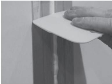
FIGURE 18: REMOVING EXCESS SEALANT
