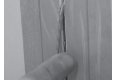
FIGURE 12: REMOVE EXCESS ADHESIVE
