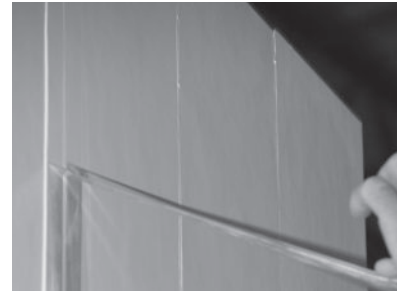
FIGURE 20: REMOVING PAINTERS TAPE
