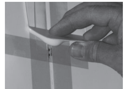
FIGURE 17: APPLYING THE PAINTER TAPE HORIZONTAL IN 3' SECTIONS
