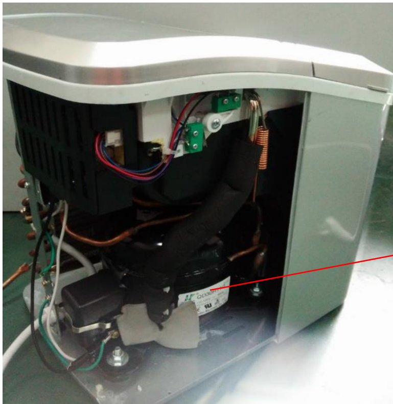
Photo 14 - Alternative compressor QD30H11G manufactured by Anuodan
