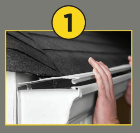
Clean gutter and place the Armour Screen on the gutter with the flat edge towards the house.
