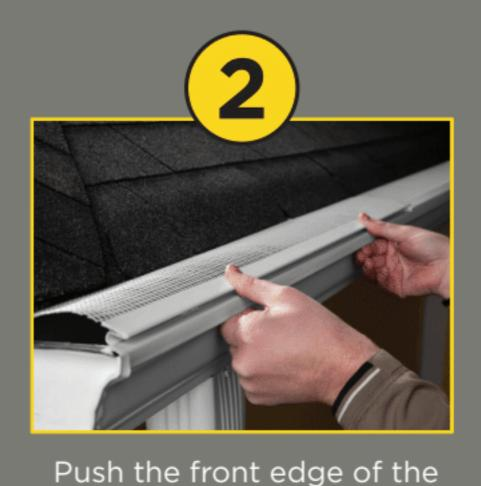
Armour Screen towards the front lip of the gutter, the C-Lock Clip will snap into place. The back edge of the screen should be pushed down and even with the back of the gutter. Some upward bowing in the middle of the screen is normal. If the screen is bowing downward, please remove the screen and try placing it again. Continue installing the screens until you reach the end of the gutter. Cut the last piece to size
