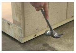
(55) Attach bottom edge of siding to floor, using an 8" to 12" nail spacing. Do not leave the back wall standing alone for a long period of time, without firmly bracing it.
