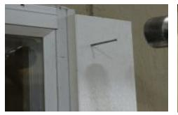
(137) Align side trim piece along the lines on the window frame as shown and attach using 2" trim nails. Repeat for the left trim piece.
