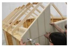
(101) Install the piece towards the front first, making sure it is aligned with the rafter and the chalk line. Note: Grooves in gable siding should align with grooves in wall siding, as shown in next step.
