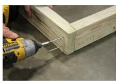
(8) Attach the band board, using 3" screws, through the pre-drilled holes.
