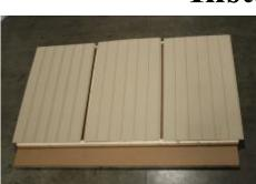
(32) Lay out siding as shown here, with the overlap towards the left.
