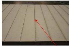
(40) Nail along the splice, making sure the splice is parallel, and looks similar to the other grooves.
