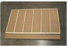
(31) Attach top plate, using 3" screws.
