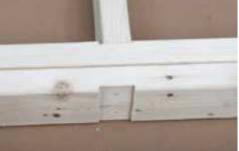
(30) Before fastening the double top wall plate, ensure that dado grooves align with wall studs, and are faced outward.
