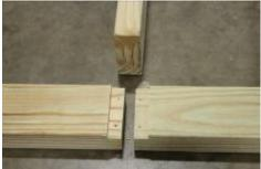
(5) Note: The band boards have dado grooves precut to ensure proper joist placement.
