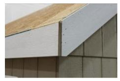
(133) Completed! Repeat on the other three corners. Note: This is the best time to paint the shed; before the windows, shingles, doors, corner trim, and vents are on.
