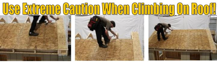
(122) Pull gable overhang parallel with the roof sheathing, then attach along gable rafter, using 2" nails every 8 to 12 inches.
