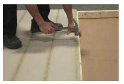
(37) Ensure that stud is parallel with siding, before nailing. Then firmly attach siding section along all edges and into each wall stud, using an 8" to 12" nail spacing.
