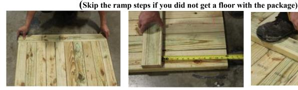
(167) Lay out the ramp pieces, if you got a floor with this unit. Note: You will need to cut one 6' board in half for the cross pieces.
