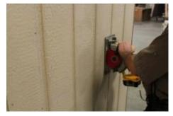
(88) Remove the screws and chalk line, then; set the saw at 1/2", and cut along the lines.
