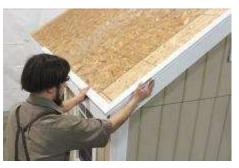
(172) Overlap the gable piece over the bottom piece and nail only the bottom.
