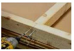
(28) Repeat the process for the rest of the wall studs; but use four 3" screws as shown, for any splice.
