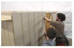
(82) Nail siding along top edge, making sure the siding is parallel with the center of the double top plate.
