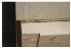
(34) Nail this corner with one 2" nail, before moving to the next step.
