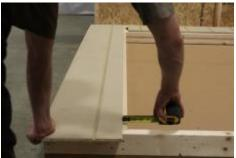
(64) Make sure siding has 3/4" reveal along edge of door frame. then nail along door frame. Finish nailing this piece.
