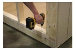
(77) Fasten to floor, using 3" screws, every 12 to 14 inches, trying to hit the floor joist.
