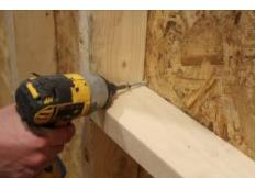
(86) Run a 2" screw through siding at each corner of the window.
