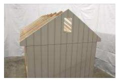
(103) Repeat with the rest of the peak pieces, making sure the bottom is flush with the chalk line. Repeat the process on the other gable, again; making sure overlap is towards the front.
