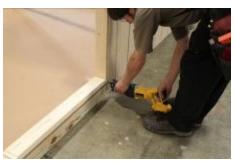
(72) Cut out bottom plate at door opening, using a sawzaw.
