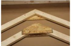
(90) Lay out the rafter pieces and the gussets. Note: Two rafters will be assembled using only one rafter gusset, the remaining rafters will be assembled using two rafter gussets.
