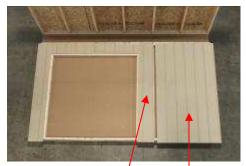
(67) Fasten the piece on the right side of door, using the same steps as the left side of door. Before fastening the last piece, check if the door opening is square. IF NOT, pull the bottom of the wall left or right to adjust it, then fasten the last piece.
