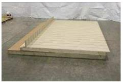
(49) Fasten the rest of the soffit much the same way as the siding. Last soffit piece should overhang by 1/2"as well. If necessary, cut to fit.
