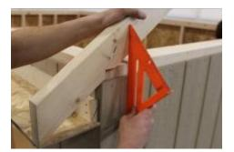
(95) Screw rafter to top plate, using a 3" screw, making sure rafter is flush with the wall siding. Repeat for opposite end of rafter.
