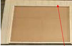
(66) Repeat with the next piece, making sure the siding has a 3/4" reveal on the top of door, as done in previous step.
