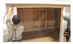
(144) Repeat for the other side, making sure the trim to trim opening is 72" before nailing. Check the measurement on the middle and bottom as well.
