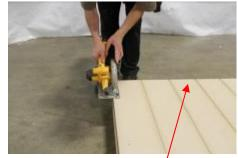
(43) Set the saw to 1/2" and cut along the line so that it is flush with wall frame.IMPORTANT! Do not cut along the bottom of wall.
