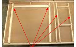
(57) Front wall is done much the same as the back wall except for the door and window studs. Locate double studs with dado for the door, and single studs with dado for the windows.
