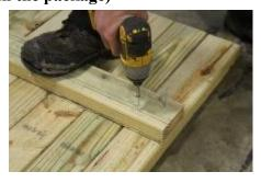
(169) Attach crosspieces to ramp boards, using two 2" screws per board. Countersink the screws approximately 1/4"
