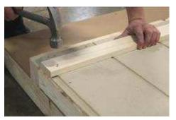
(46) Align bottom of 1x3 soffit strip with chalk line, and keep flush with wall frame, then secure, using 2" nails, and nailing on every stud.
