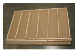
(26) Be sure to alternate top wall plate splices.
