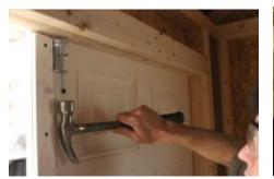
(155) Pull door in, tight against the frame, then make a mark for the inside latch pin. Repeat on the bottom.
