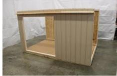
(69) Set the front wall, again: making sure edges of wall are flush with edges of floor. It is <u>VERY</u> important that a person holds the wall in place until wall is attached firmly to floor, or braced.
