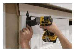
(151) Start with the left door, and fasten to trim using 2-1/2" black screws, and making sure you keep the top of the door down from the trim, approximately 1/4".
