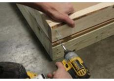
(27) Insert two 3" screws through the pre-drilled holes to attach bottom plate to each wall stud. Make sure bottom plate and wall studs are flush.
