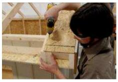
(106) Fasten gable overhang to rafter, using 2" screws, every 8 to 12 inches.
