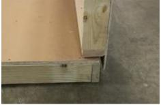
(51) INCORRECT! Wall needs to be flush, and in against the floor frame, and down against the flooring.
