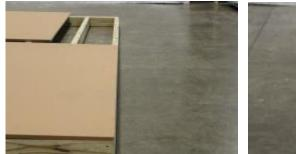
(16) Nail along the gable, again; making sure flooring is flush with the floor joist. Use an 8" to 12" nail spacing.
