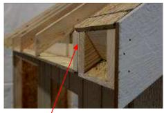
(105) Make sure the gable overhang is flush with the rafter, and tight in against the gable siding, as shown.
