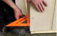
**(84)** Correct! Attach to wall studs, using 2" siding nails.
