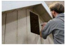
(139) Install vents, caulking around the perimeter, before installing.
