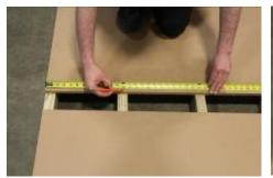
(22) Before you finish attaching the first row flooring to the joist, make marks 12" on center for a guide to adjust the joist when nailing.
