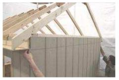
(100) Snap a chalk line 1/4" below the bottom of the soffit as shown.
