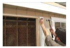
(143) Align trim flush with edge of siding and attach, using two - 2" trim nails spaced every 12 to 14 inches.
