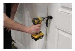
(158) Install latch using 2" black screws.
