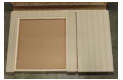
(62) Lay out siding as shown here, starting with the under lap towards the right.
