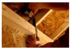
(164) Install hurricane ties, using 1-1/4" screws.
