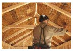
(163) Fasten the crosstie, using 3" screws. Note: Divide the crosstie out equally.
