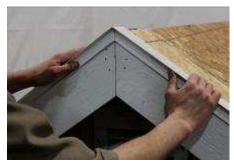
(175) Bend around the top as shown. This top piece should overlap the bottom piece. Do not fasten it till the bottom piece is installed on the other side. Finish installing the rest of the drip edge.
