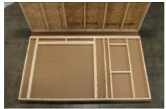
(61) Fasten the other studs, using the same pattern as the back wall.
