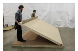
(50) Set the wall, making sure edges of wall are flush with edges of floor. Note: It is <u>VERY</u> important that a person holds the wall in place until wall is attached firmly to floor, or braced.
