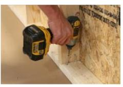
(54) Repeat for the rest of the wall, again; making sure wall is in against the floor frame.
