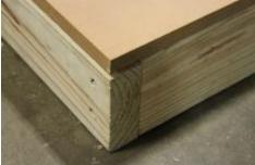
(14) Start on the front corner with a full 4'x8' piece, making sure flooring is flush with floor joists.
