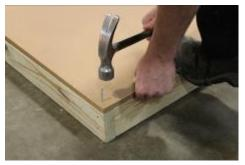
(15) Attach the corner of the flooring, using 2" nails.
