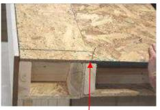
(118) Starting with the left piece, push roof sheathing tight against the gable overhang, and align flush with bottom edge of gable rafter, then attach, using a 2" nail.
