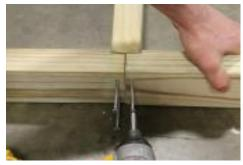
(9) Screw the rest of the bandboards into floor joists. Important! Band board splice needs to be tight.
