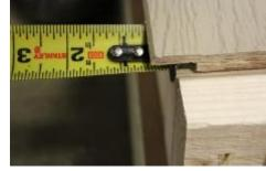
(33) Place the siding even with the center of the double top plate, and 1/2" out over the wall stud.
