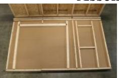
(56) Locate and lay out the parts to assemble the front wall. Note: Front wall plates have extra dados for the door and window.
