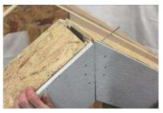
(109) Incorrect! Before fastening the overhangs on the top, make sure the splice is uniform, as shown in next step.
