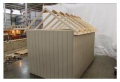
(97) Install the rest of the rafters, 24" on center, or in every dado groove on the top plate. Repeat, till all rafters are installed.
