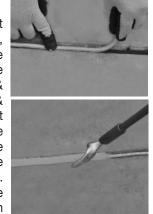
wrapper will liquify immediately, continue to move the flame back & forth, side to side, in a slow even manner, heating about one foot at a time. The stix will start to liquify immediately but you should continue heating for about 1 - 2 minutes. The type of torch, along with wind, temperature conditions, and thickness of stix will affect melting time. Traffic Ready in approximately 20 minutes.
