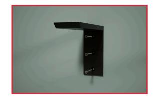
3. Once your brackets are in place and level, using the holes on the bracket as a guide, drill pilot holes into your wall studs. With your pilot holes now made, fasten your brackets with by screwing them to the wall.
