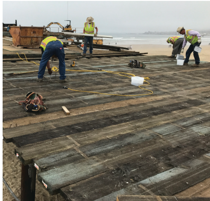
Pier restoration in progress.
