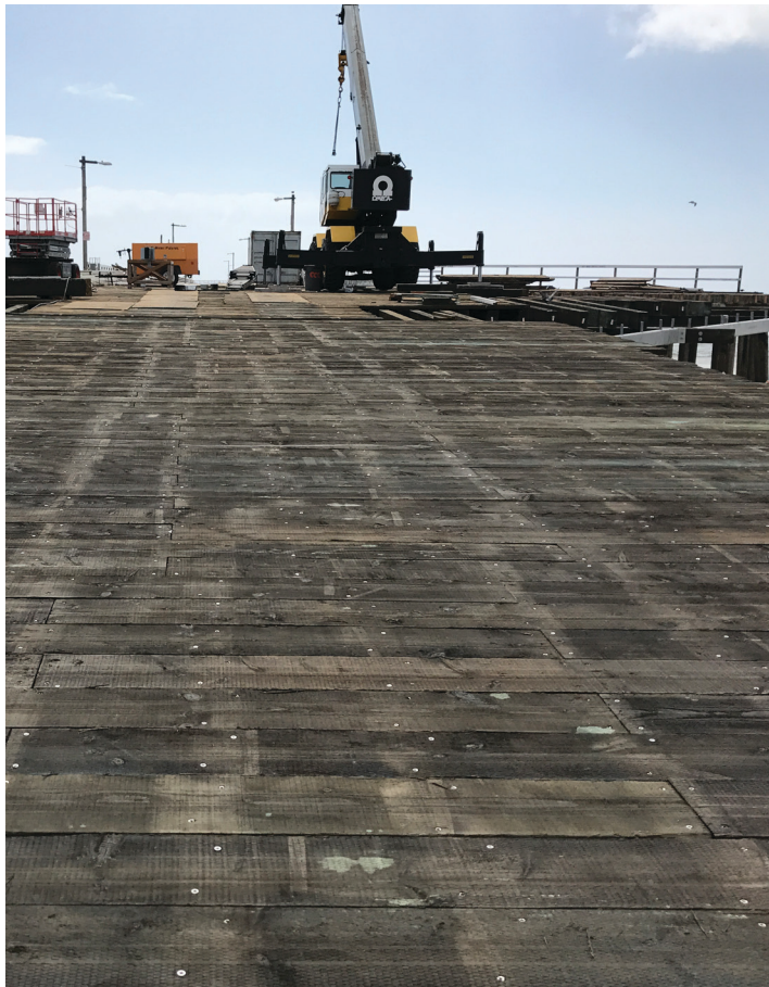
Newly installed pier deck boards.
