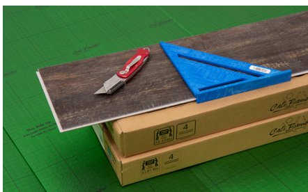
Cutting boards using Score and Snap technique
