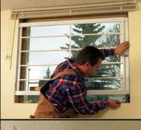
**07.** With window bar level, mark position of screws.
