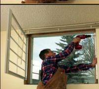
**08.** Pre-drill the holes for the screw and fasten with 1 3/4" screws.
