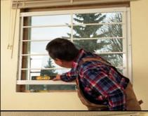
**06.** Position **RIGHT GUIDE RAIL** on right side of window and check level. (NOTE: For HINGED MODELS position RIGHT GUIDE RAIL plus LOCK END BRACKET)
