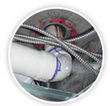
Commonly observed field devised methods may result in providing a dangerous pathway for water, smoke, gas or fire. HYDROFLAME\*\*
