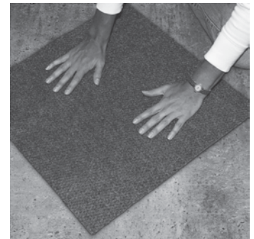
Press down firmly in desired location. This will lock the tile in that position. Continue to place tiles in desired pattern, rotating 1/4 turn. It's that easy!
