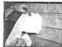
Position LintCatcher over the vent
