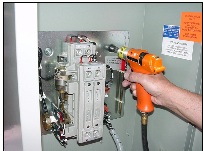
Figure 7-7 Installing the Contactor
