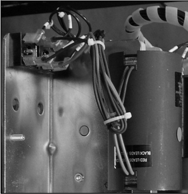
Figure 7-91 Rectifier Connections and Tie Wraps
