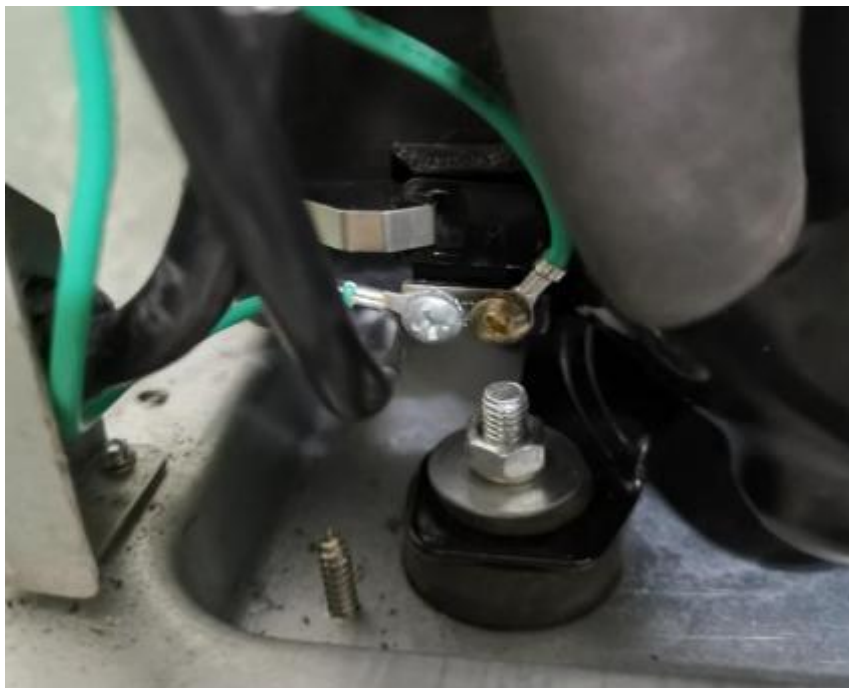
Photo 4.14 - Earthing terminal view for HZB-**N, **NA, **NB, **AN, **BN, **CN, **DN series model
