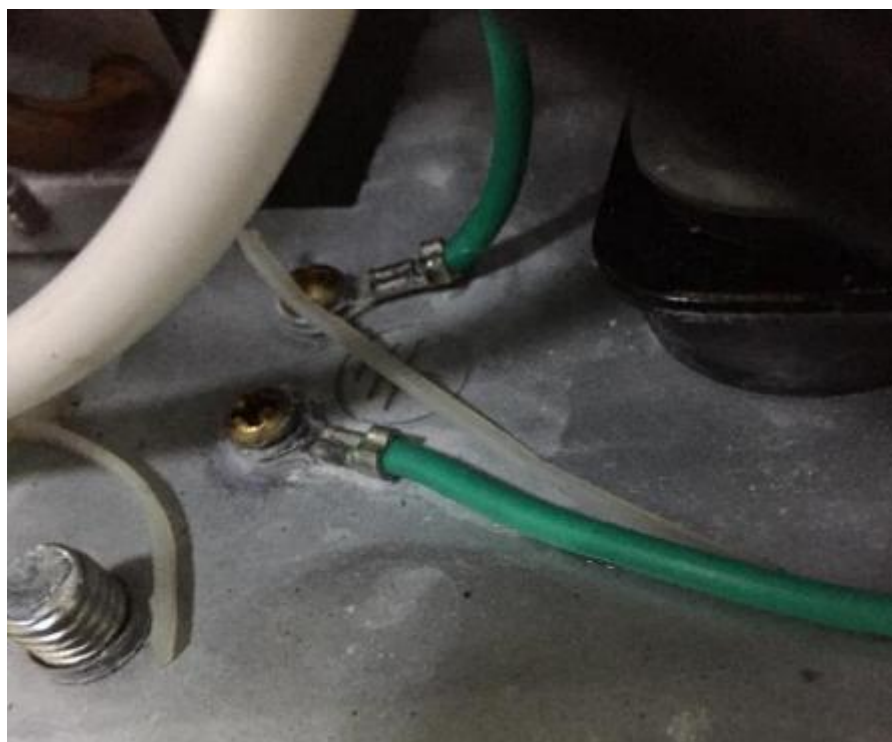
Photo 3.12 - Earthing terminal view - HZB-30D
