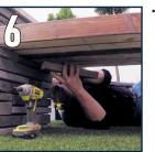
Using a **Drill** and **2.5 in. screws**, affix the sections of trimmed wood to the bottom of the boards to prevent sliding.
