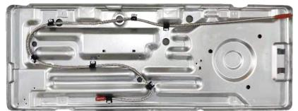
"BHI" Outdoor Unit has "Heating Belt" that works by Temperature Sensor, if temperature lower than 32°F (0°C) degree, it would start to heat and when over than 32°F (0°C) degree, would stop working automatically to ensure that Outdoor Unit does not freeze, it's a great feature to use BHI Mini Split AC at cold temperature region / area / season.
