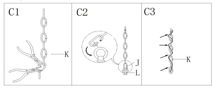
Step C1: By measuring, determine the correct number of links needed for proper hanging height. Using the chain pliers, disconnect and discard the remaining chain.
