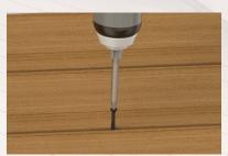
5. With the new board held firmly in place, fully tighten down the screws of each Grip-Rite® Ninja® Hidden Deck Clip. Set the drill to 1/3 of the Max torque. If your drill has the option of a clutch mode, it is recommended you use that. Impact drills should not be used with Grip-Rite® Ninja® Hidden Deck Clip.
