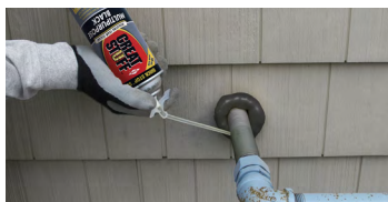
Around gas lines
