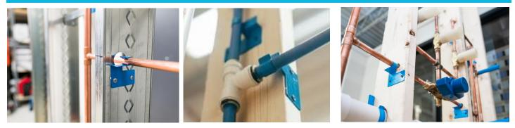
Inside of the wall: For applications that need to go through the center or back of the stud
