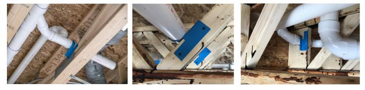
Outside of the wall: For applications that need to go through trusses or the back of joists
