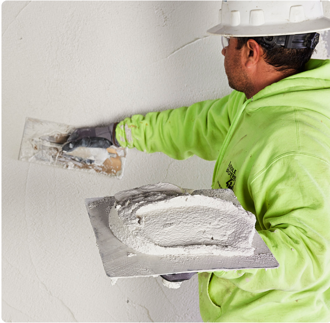
Base (first) coat on Kal Kore Plaster Base
