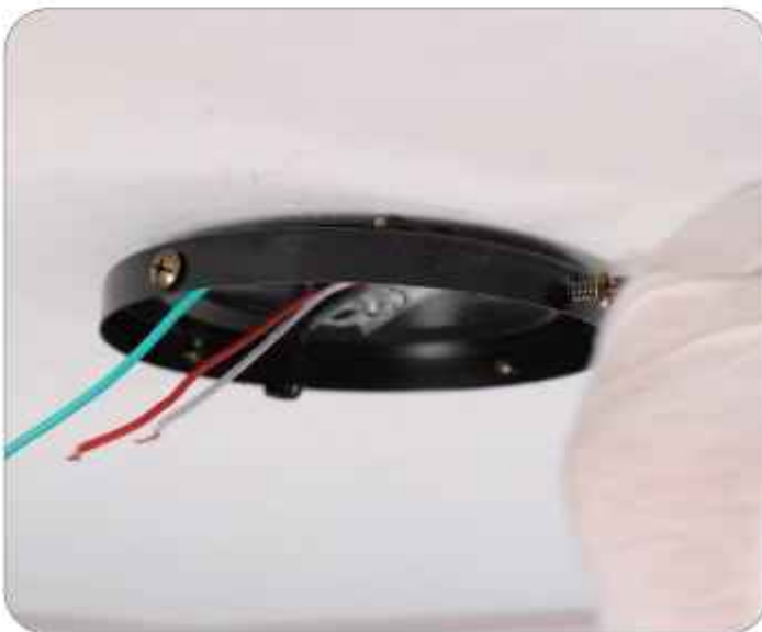
11. Loosen the screws
