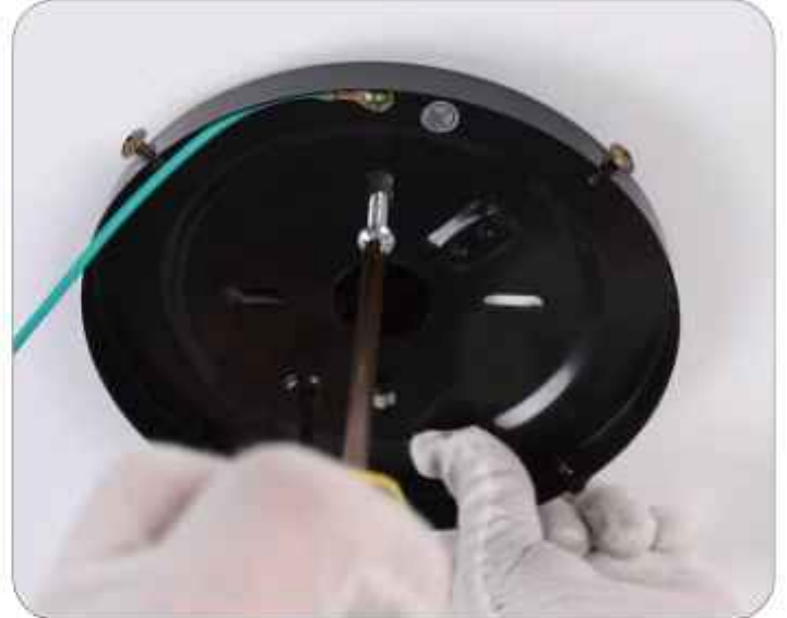
10. Tighten the screws to secure the hanger
