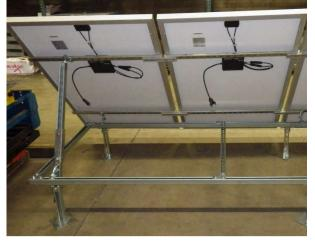
9. Then the "A1 & A2" AND "A3 & A4" will be connected using the splice bar (flat 4 hole plate in the box). There are two splice bars given in the box with hardware.
