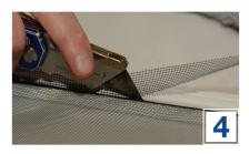
Use utility knife to trim excess spline and screen from frame, making sure to cut toward outside edge of spline groove to prevent damage to the newly installed fabric.
