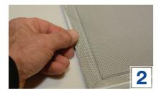
Lay screen fabric over frame, align squarely and overlap 1/2" on all sides.
