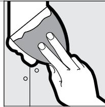
Apply an even coat of all purpose or taping compound over the length of the joint with a 6 in. knife.
