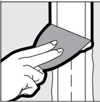
Remove excess joint compound from edge and apply a thin coat over the tape. Allow first coat to dry overnight. Scrape off bumps, ridges and other imperfections with knife. Be careful not to damage.
