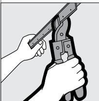
Trim length 1/2 in. shorter than the wall height by cutting through each flange with metal snips, then bend and snap. Hold metal cornerbead firmly against corner and mechanically fasten through small holes every 9 in. on flange.
