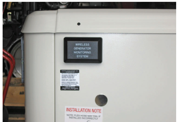
Figure 3 — Mount Transceiver
