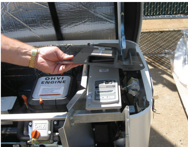
Figure 1 — Remove Control Panel Cover
