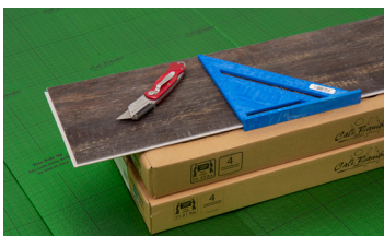
Cutting boards using Score and Snap technique
