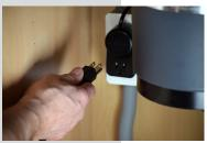
Step 2 Unplug the disposer from the single outlet power module.
