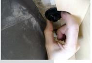
Remove plastic nut from air transmitter body underneath the countertop.
