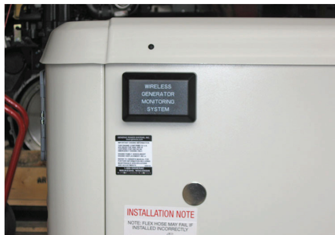
Figure 3 — Mount Transceiver
