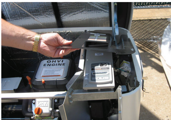
Figure 1 — Remove Control Panel Cover
