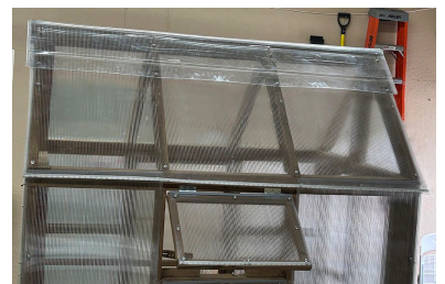
Ridge Cap: Exterior View
