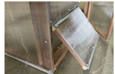
Front Window: Exterior View
