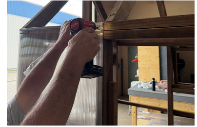
Front Wall Panels: Pre-drill Holes
