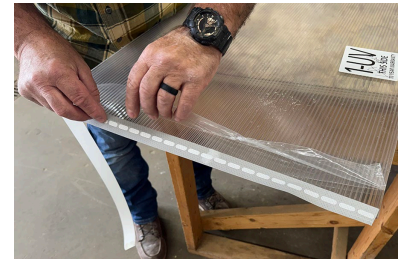
Edge Sealing: Anti-Dust Vent Tape
