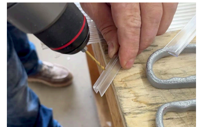
Attach U-Channel: Drill Weep Holes
