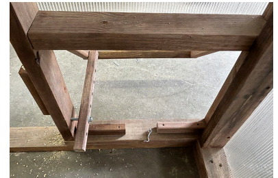
Front Window: Interior View
