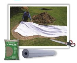
With the pond excavated you now need to add a barrier to protect the liner from potential punctures caused by stones or plant roots.
