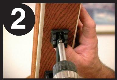
Insert stem in foot and attach pivoting head to handrail.
