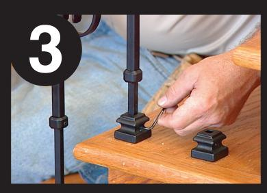
Tighten adjustment screws to lock baluster in place.
