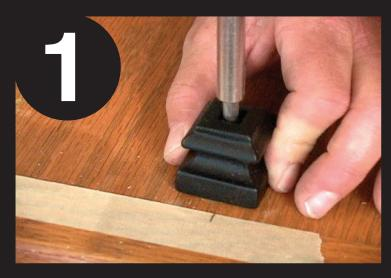
Attach shoe of baluster to step at desired location.
