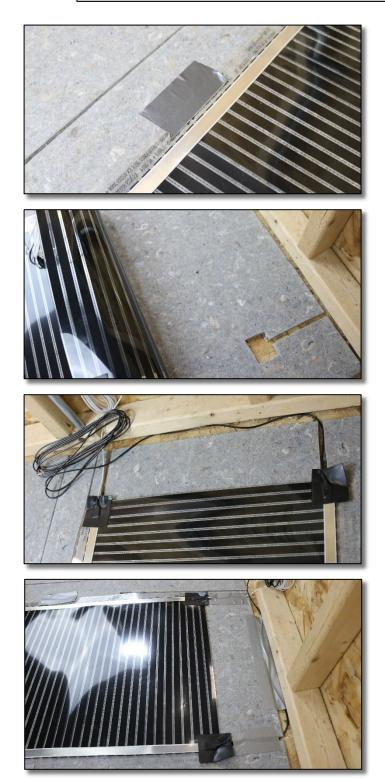
Lay the mats out according to your design plan and tape in place with a high quality duct tape on the sides. This step is just to hold the mats in place while you continue working in the area. You don't need to tape on the ends. There is no "top" or "bottom" to the mats.
