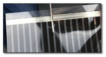
Make a cut across the silver metal conductor bar one black heating element from the end of the mat. Do not cut into black heating element bar as this will cause the GFCI to trip.
