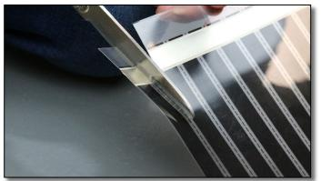
Cut through the last black heating element bar to remove the end of the silver bus bar, creating a notch. Do not over-cut into the next black bar. Repeat on both sides.
