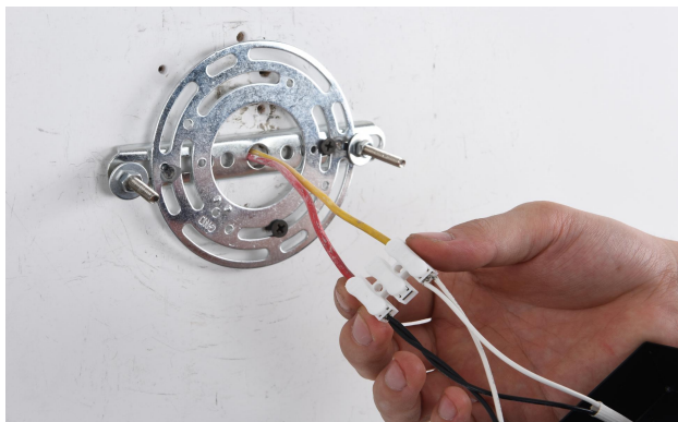
Step 3 : Install the hanging bracket and connect wire
