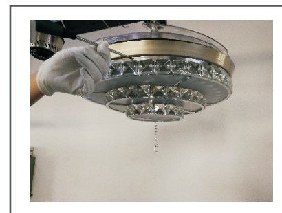
Step 8. Install and fix the lampshade on the chassis with screws.
