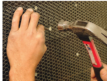
Install corrosion resistant metal lath.
