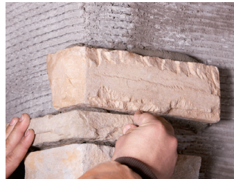
Install corner stones first.
