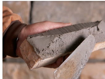
Apply mortar to the entire back of the stone.
