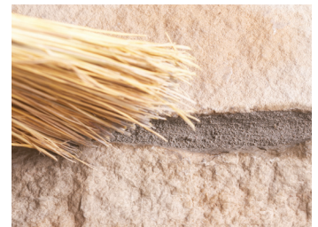
Brush off excess mortar with a dry brush.
