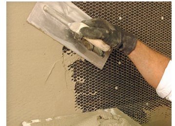
Apply mortar for scratch coat.
