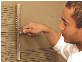
Rake mortar to create scratch coat. Allow to dry.
