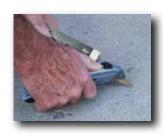
5. Gun Slab into the crack. For wider cracks (1" wide or more), apply 3 beads: 1 on each side of the crack, and another down the middle. This ensures enough product is in the joint, and makes tooling easier.
