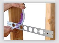
Position #704 until bracket fits into groove, then rotate into place.
