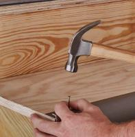
Place Vinyl Plank Stair Nosing into position on the substrate and press down firmly for a strong adhesive bond. MAKE SURE TO CLEAN OFF ANY EXCESS ADHESIVE FROM THE VISIBLE SURFACE OF THE STAIR NOSING AND VINYL PLANKS.
