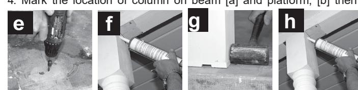
from beam to platform [c] for each column. If necessary, trim post to length (cut only the top). If trimmed, the top of the column must be primed again using high-quality acrylic primer.
