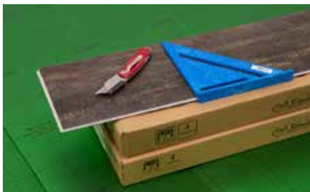
Cutting boards using Score and Snap technique
