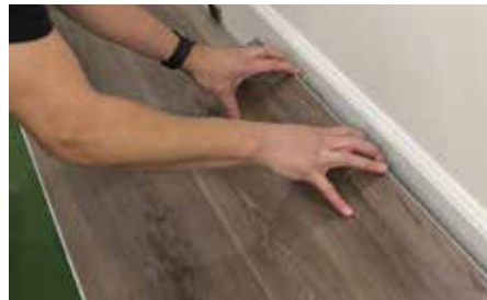
Diagram A For row three onwards, installation does not require alternating rows.
