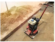
Use a vibratory plate compactor or hand tamper to compact the freshly excavated subgrade material. Add paver base material in 2" layers, spraying with water to keep moist while compacting. Repeat process unil final thickness of base is reached. (approx. 6" (152.4mm))
