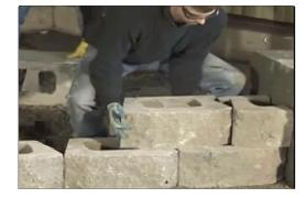
Begin placing the second course of block at straight wall areas being sure to center each unit over the joints of the blocks below in a "running bond" or 1 over 2 pa ern.
