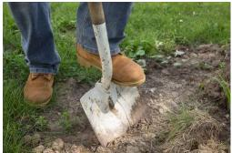
Visit www.call811.com before any digging or excavaon. Dig a trench approximately 10"(254mm) deep by 16"(406.4mm) wide to your desired length and shape (straight and/or curves) being sure to remove large rocks, roots, organic material, etc..
