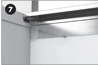
Pre-drill holes w/ 1/16" bit & attach the
